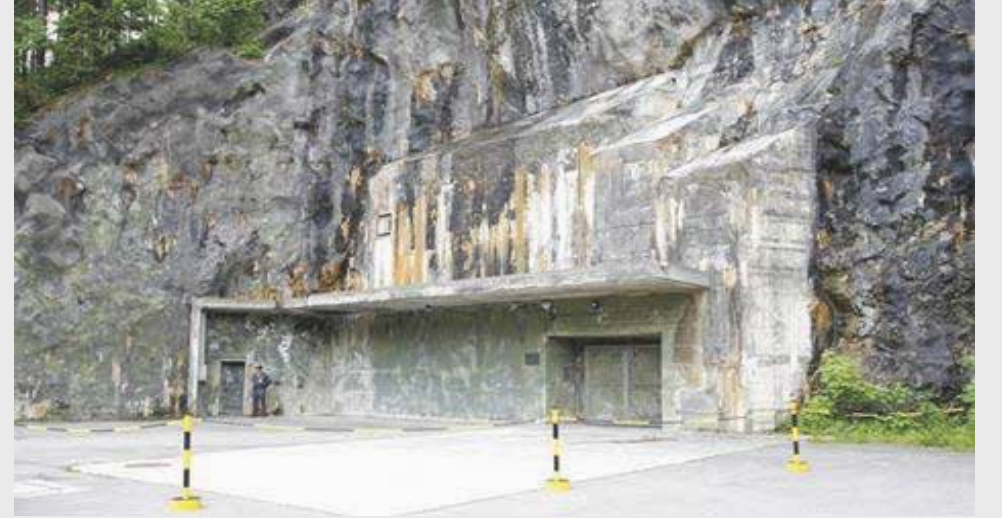
Görsel Kaynak: Data Center Knowledge. (2010, November 8). Closer Look: The Swiss Fort Knox Data Bunker.
