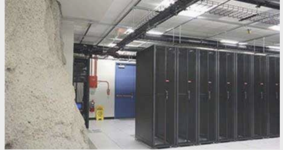
Görsel Kaynak: "Bluebird's Underground Data Center Provides Innovative Construction and Location Benefits." Bluebird Network
